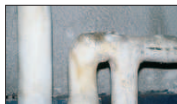
© INRS Calorifugeage
