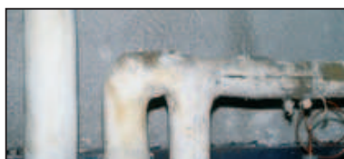
© INRS Calorifugeage
