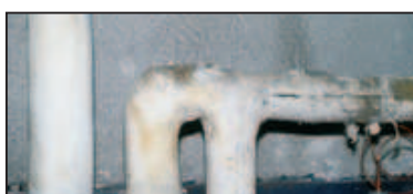
© INRS Calorifugeage
